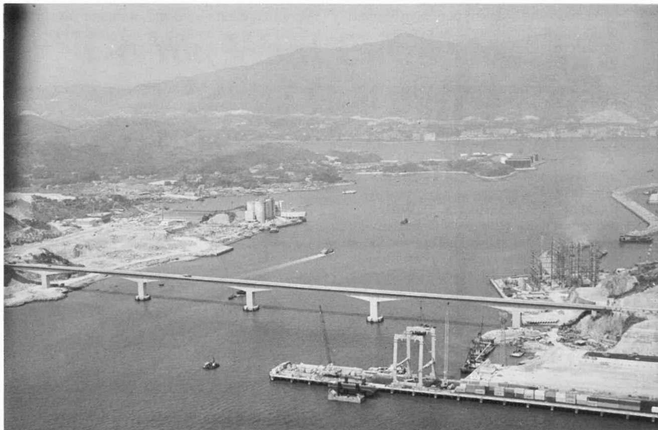
The Tsing Yi Bridge, longest in South East Asia, was partially financed by American oil companies
